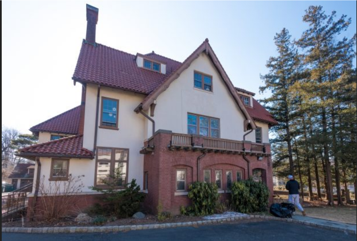
The Montclair Sanctuary Project at Bnai Keshet, a team of about a dozen volunteers from a variety of religious institutions complete repairs and painting Saturday Feb. 3 to the third floor of "Red Gables" at Bnai Keshet, a shelter for immigrants in danger of deportation. ADAM ANIK/FOR MONTCLAIR LOCAL
